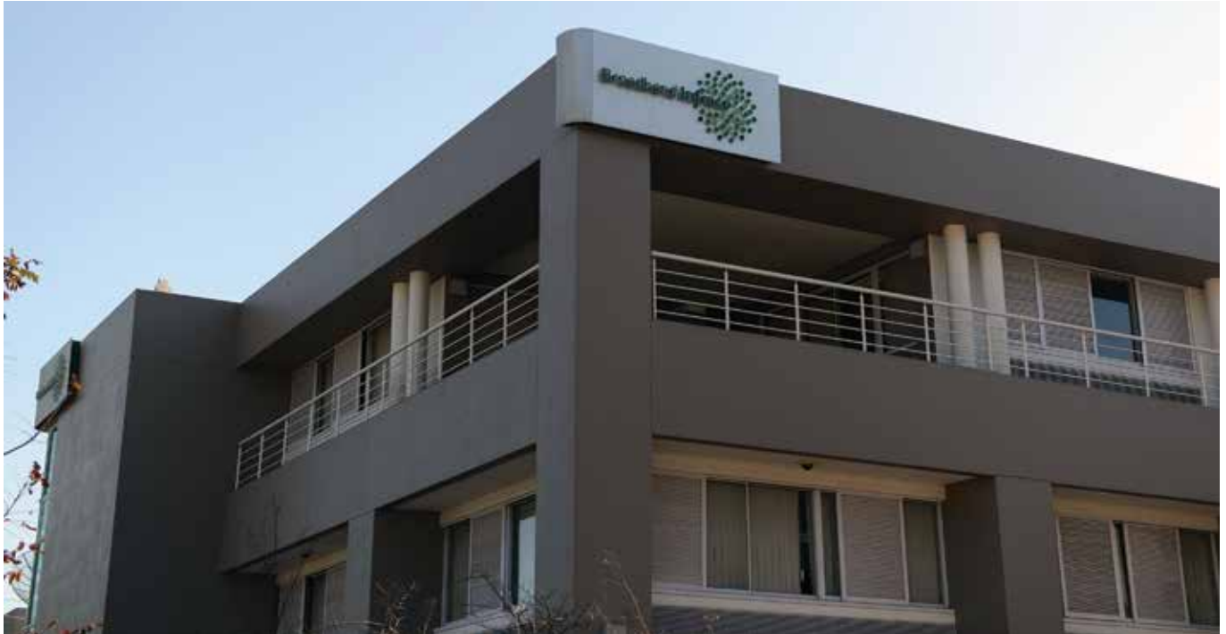
Broadband Infraco head office. Building 9, Country Club Estate, 21 Woodlands Drive, Woodmead, Sandton.
