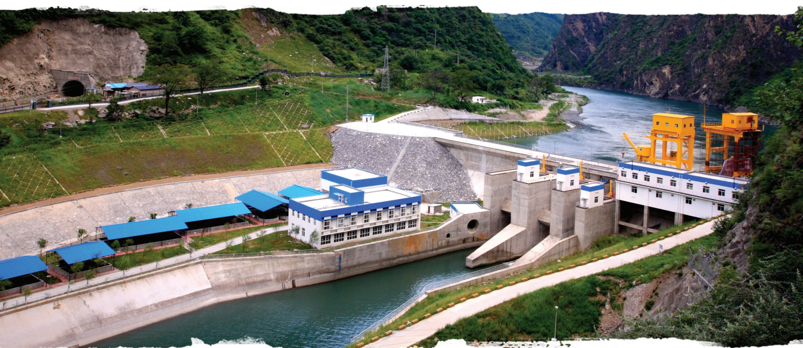
Jiangbian Hydro Power Station
