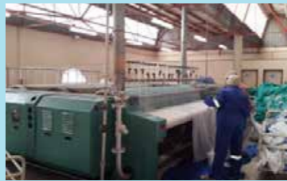
Laundry units replaced in Mankweng Hospital.
