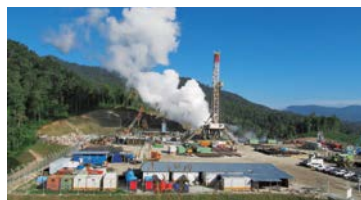
Project construction site
