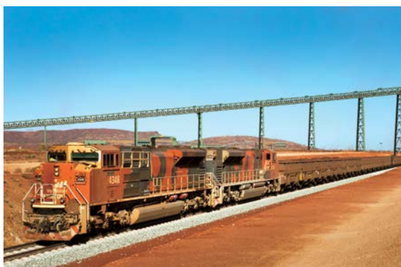
Railroad for transporting Jimblebar iron ore (photo courtesy of BHP Billiton)
