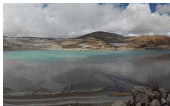
Tailings storage facility at Cerro Corona, Peru
