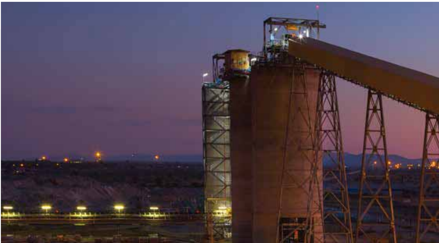
The silos and feed conveyor from the shaft at Styldrift I
