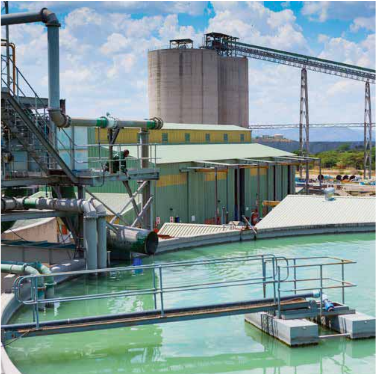
The water settling tank at the BRPM concentrator
