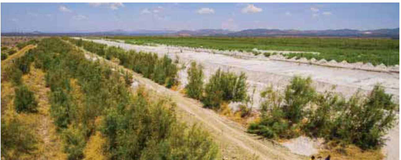
Vegetation on the wall of our tailings dam
