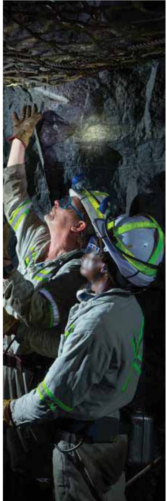
Coaching on the installation of a safety net
