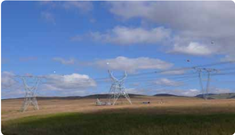
New high-voltage lines are erected from the Ingula pumped storage scheme near Ladysmith
