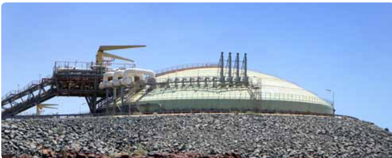
Once cooled to minus 161° Celsius, LNG is placed in specially designed storage tanks prior to shipping, such as pictured above at the Karratha Gas Plant.
