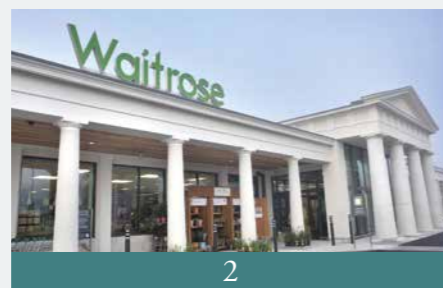
2 TRURO Eastern District Centre A partnership project with Cornwall County Council and Waitrose on Duchy-owned land.
