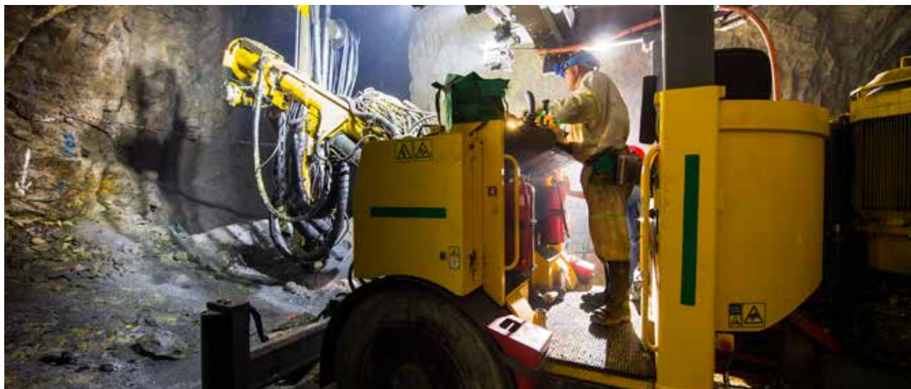
Drilling and installing support at South Deep
