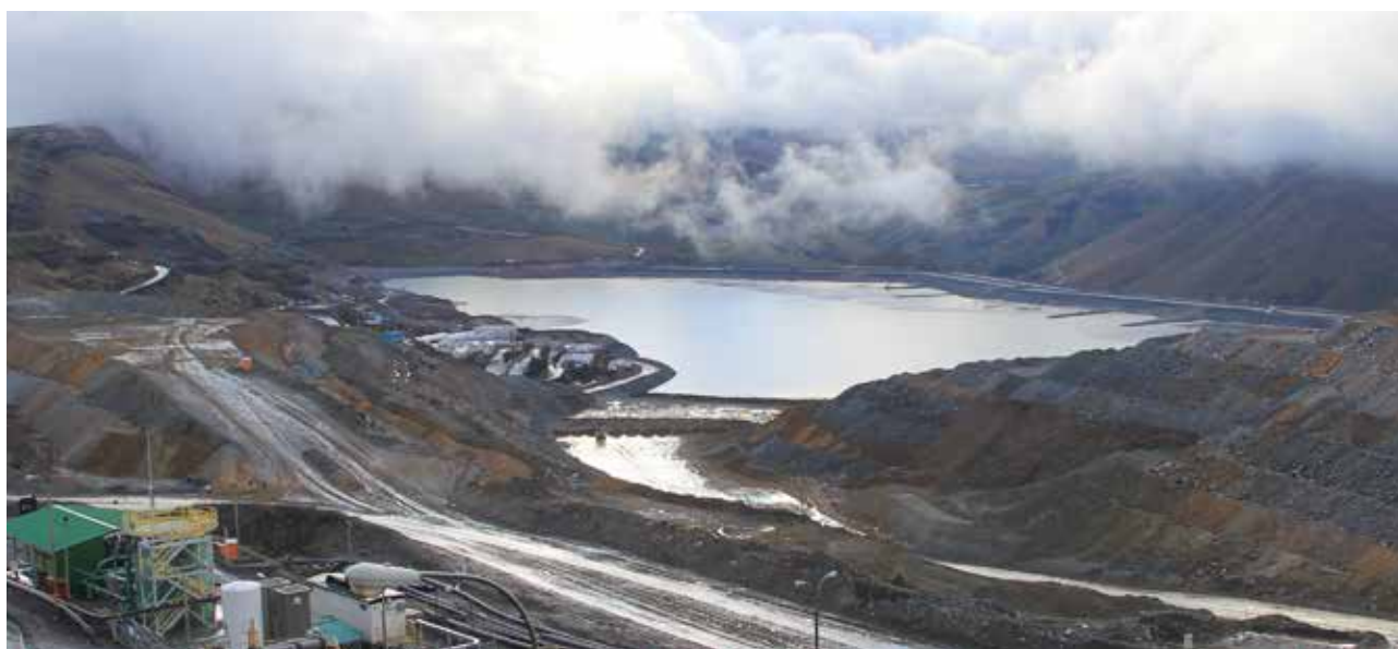
Tailings storage facility at Cerro Corona
