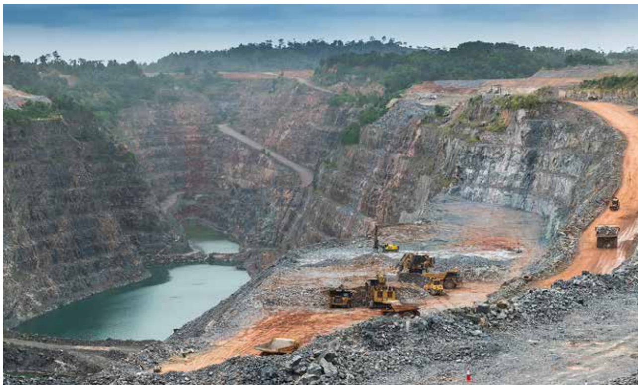
Work at the Damang pit cutback project
