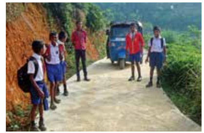
Road construction - Dessford Estate
