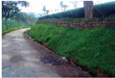
Road Banks Well Protected with Arachis Pintoii & Vetiver – Mattakelle Estate
