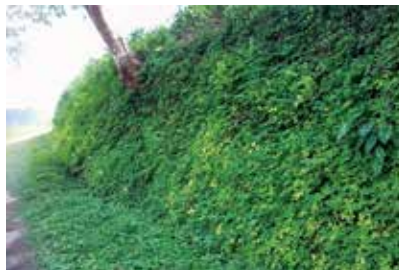
Road Banks Well Protected with Arachis Pintoii & Vetiver – Deniyaya Estate
